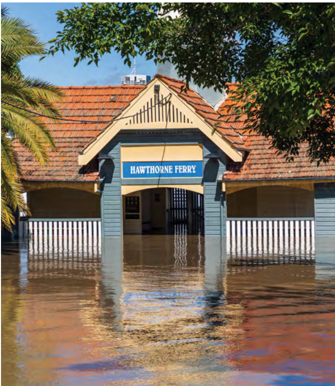
Hawthorne Ferry Terminal
