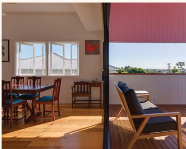
Solid sections of balustrade are an effective way of creating privacy to rear balconies, where people are typically seated. Aligning new sills to existing windows can help a renovation fit in with the existing house.
