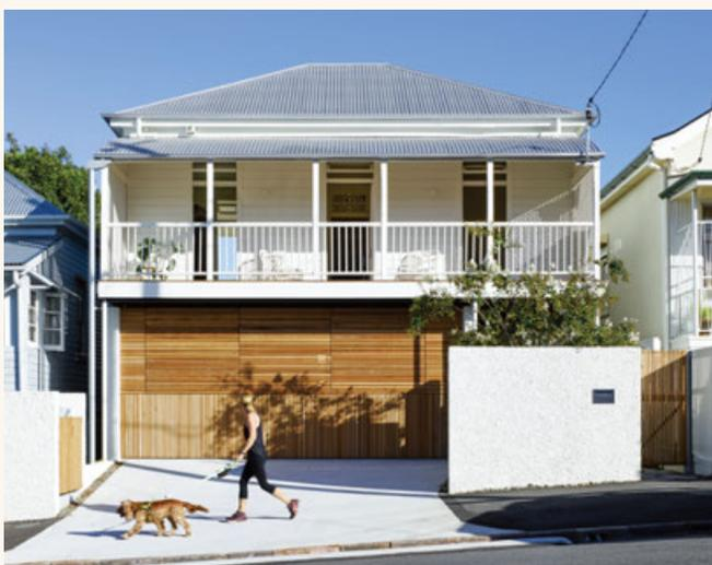
This house is an example of a narrow lot traditional home that has been renovated. The lower level, though built in, is recessed back from the verandah, to create depth and shadowing to the lower level, and uses permeable timber screens that allow air and some visibility through. The original front stairs have been removed to allow for car accommodation to fit, however the rhythm of the verandah posts and balustrade remains.
