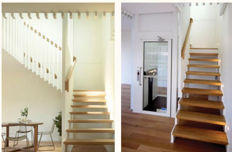
Left: Adaptability in a two storey house for ageing home occupants. The stairwell was designed with a square central light-well, at a specific size to allow for a domestic lift to be installed in future. This is just one example of how you can design flexibility and adaptability into your home.
