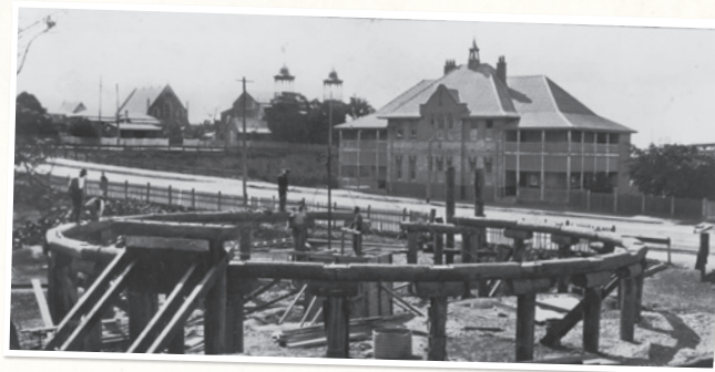
Construction of a railway turntable in Main Street, Woolloongabba, 1921, State Library of Queensland, Negative Number 37394
