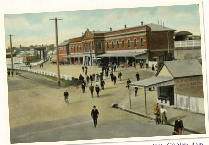
Entrance to the Melbourne Street Railway Station in South Brisbane, 1906-1910, State Library of Queensland, Negative Number APE-062-0001-0004
