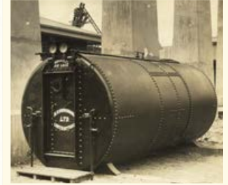
Hospital Air Lock at the Grey Street bridge construction site, 1930, State Library of Queensland, Negative Number APU-016-001-0015
