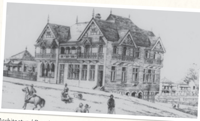
Architectural Drawing of the Normanby Hotel, Brisbane, 1890, State Library of Queensland, Negative Number 202854
