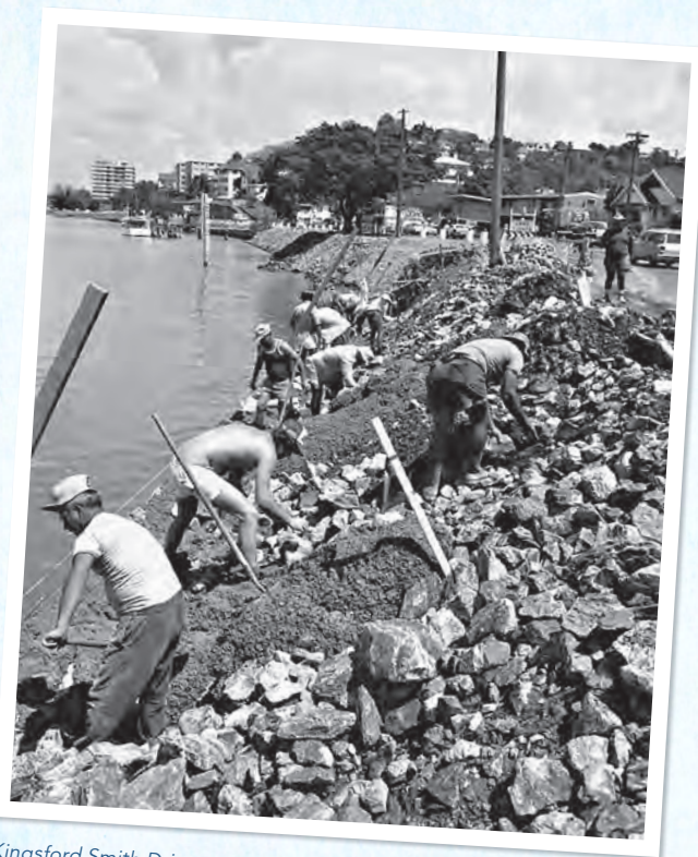
Kingsford Smith Drive road widening progress, Hamilton, 1980.
