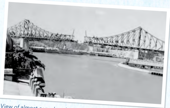
View of almost completed Story Bridge, circa 1939, image courtesy of John Oxley Library, State Library of Queensland, Neg. No. 58518.
